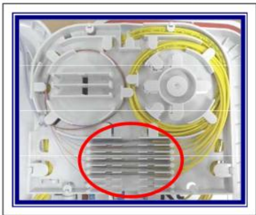
5 Step 5 to splice pigtail and fiber cable
